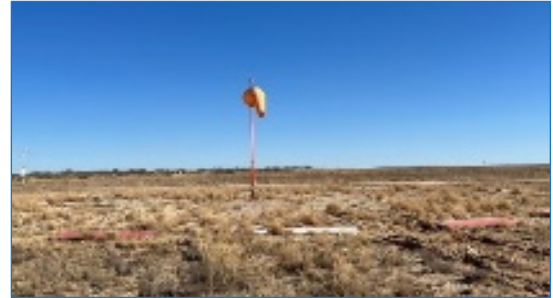
Lighted Wind Cone and Segmented Circle
